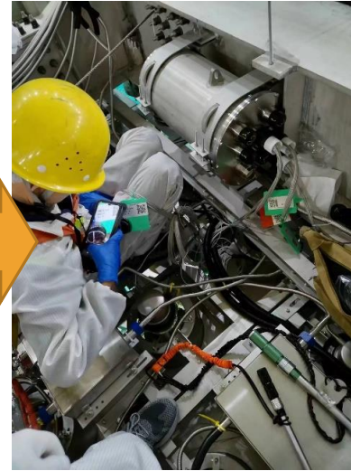
Connect SPMTs to UWB
