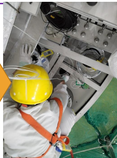
Install Light Barrier
